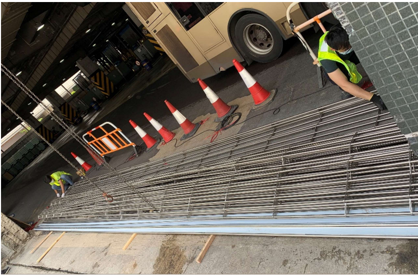
Installing Shutter curtain of Open Grille
