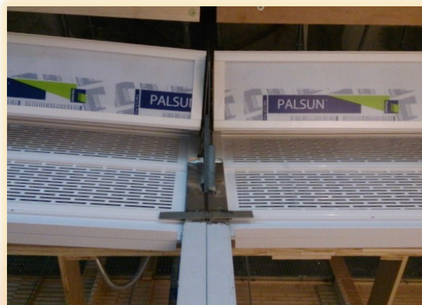
Ventilation hole; Portable Guiderail;
